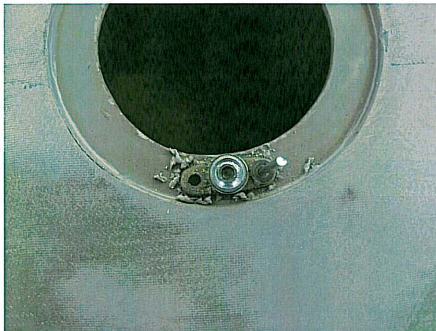
Figure 41. \varnothing 3 Hole drilling for nuts riveting, and chamfering attachment for rivet head 1 \times 45^\circ - stage 2.
