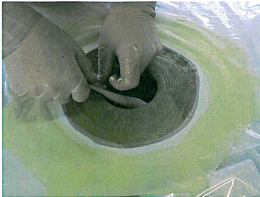
Figure 20. Placing layer 3... part 2.
