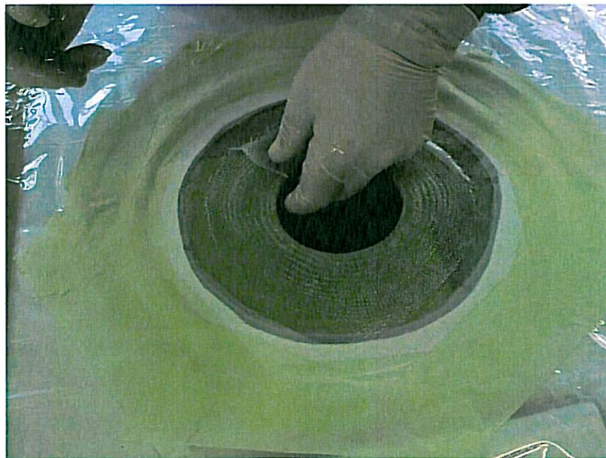
Figure 21. Placing layer 3... part 3
