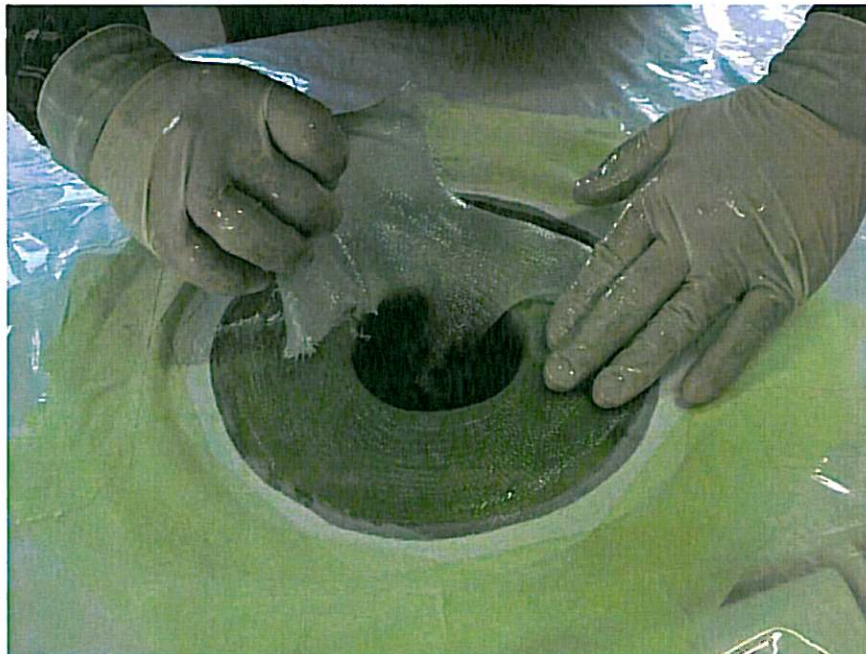
Figure 23. Placing layer 4... part 2.
