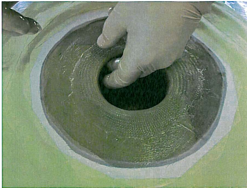
Figure 18. Placing layer 2... part 2.
