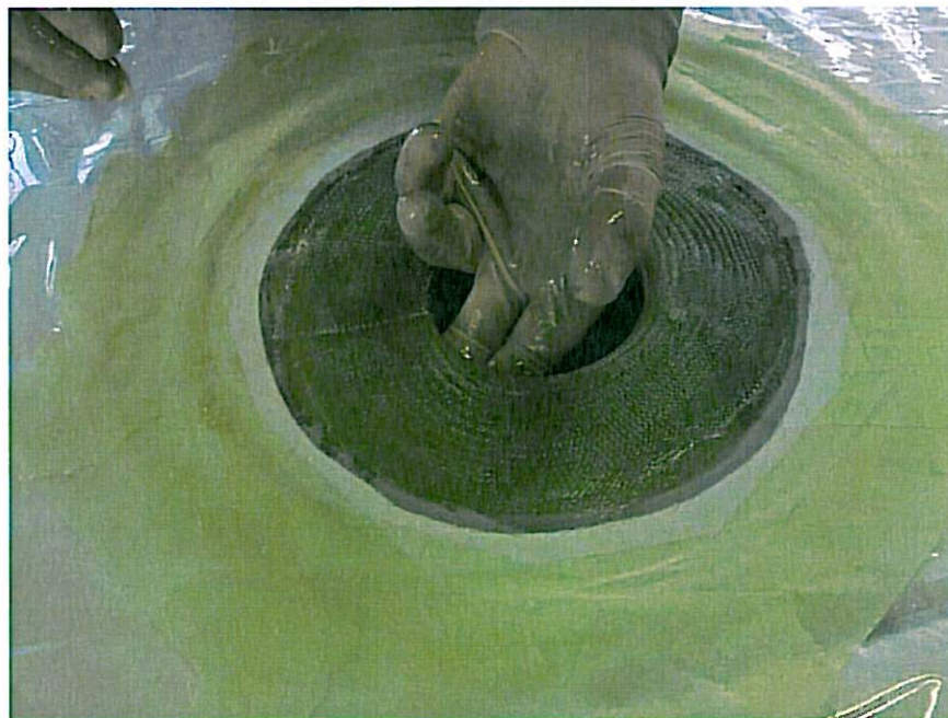
Figure 25. Placing layer 4... part 4.
