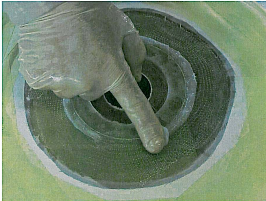
Figure 33. Removal of excess from wings outer surface.
