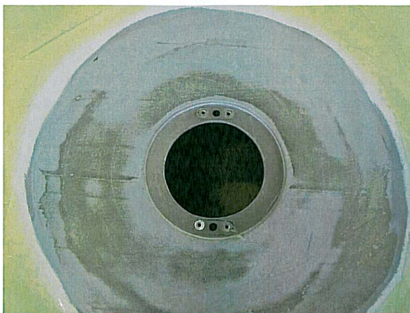
Figure 44. Repair area prepared for painting.
